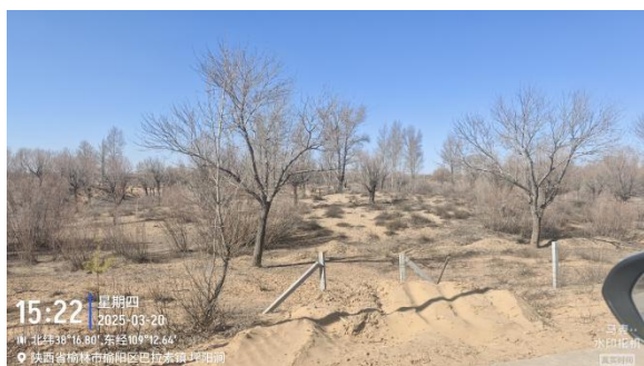
拟建地埋输浆管道沿线现状
